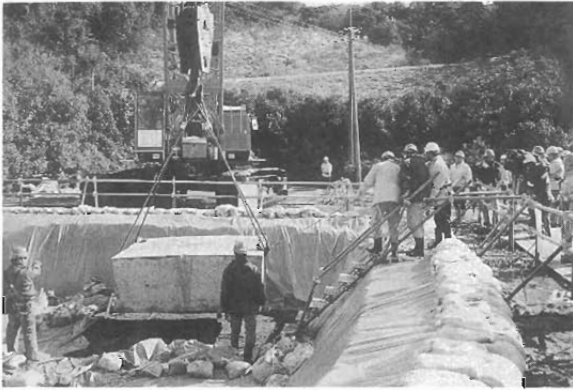
Fig.22 Burying of Outer Shield Concrete Blocks (Takahama-2)
