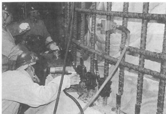
Fig.16 Welding Rein Bar (Ohi-1)
