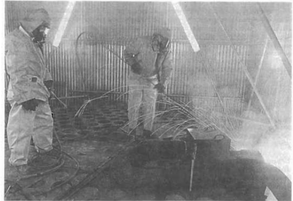
Fig.4 Top Biological Shield During Thermic Lance Process
