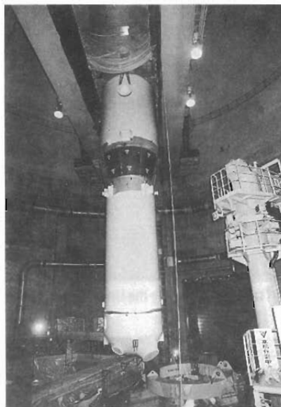
Fig.10 Hoisting SG from its Cubicle (Mihama-2)
